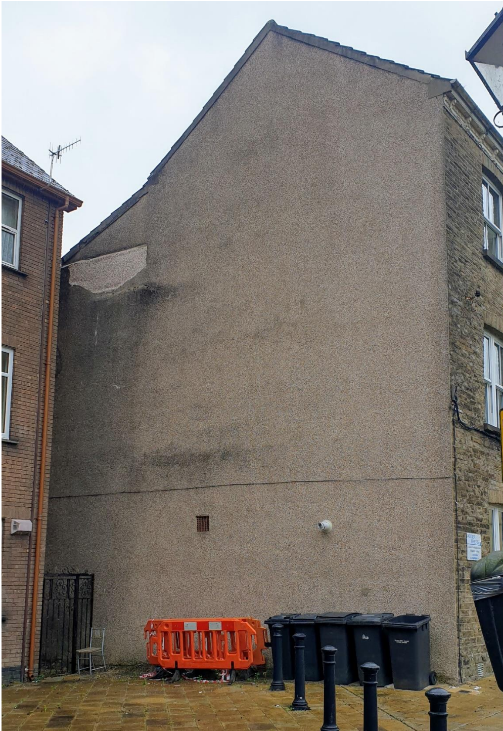
Side elevation (showing repair work)
